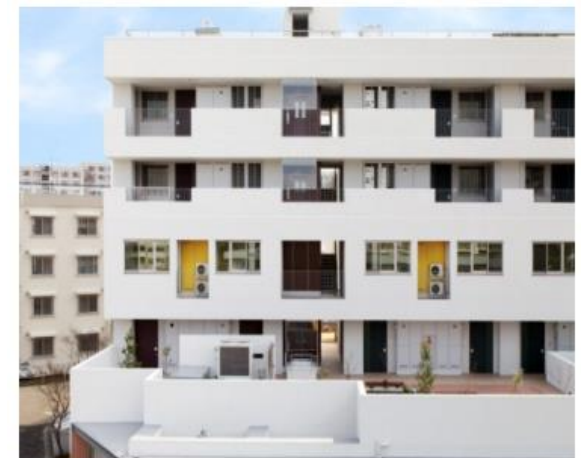
the north view
