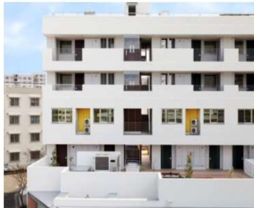
the north view
